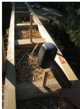
Fixing the wall plate to the bales
