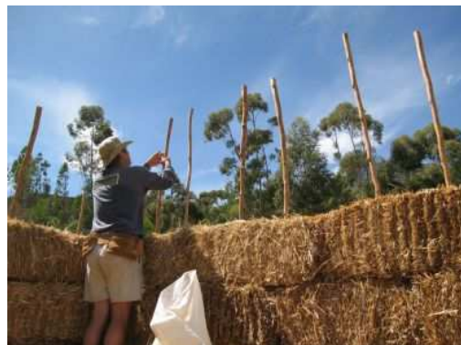
Speeding up the staking of the bales
