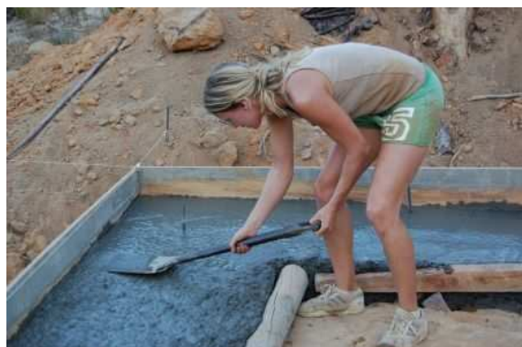
Vibrating the concrete by hand
