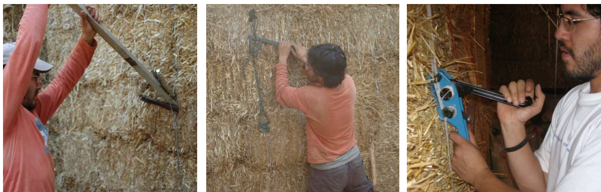
Figure 3.8: Different tie-down systems
