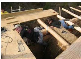
Taking out the rotting bales
