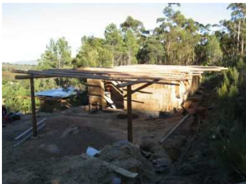
Main house with roof beams in place
