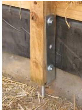
Fencing wire tie-down system
