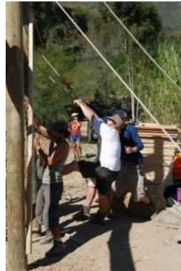
Lifting the roof beams up
