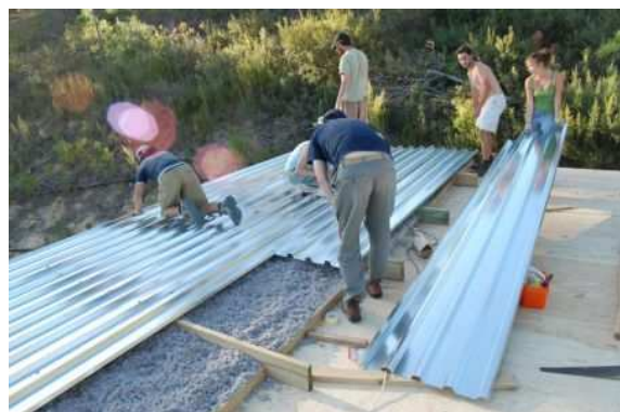
Covering the roof with corrugated iron
