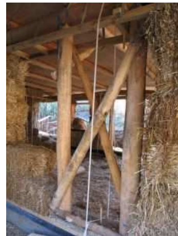
Braced columns as roof support
