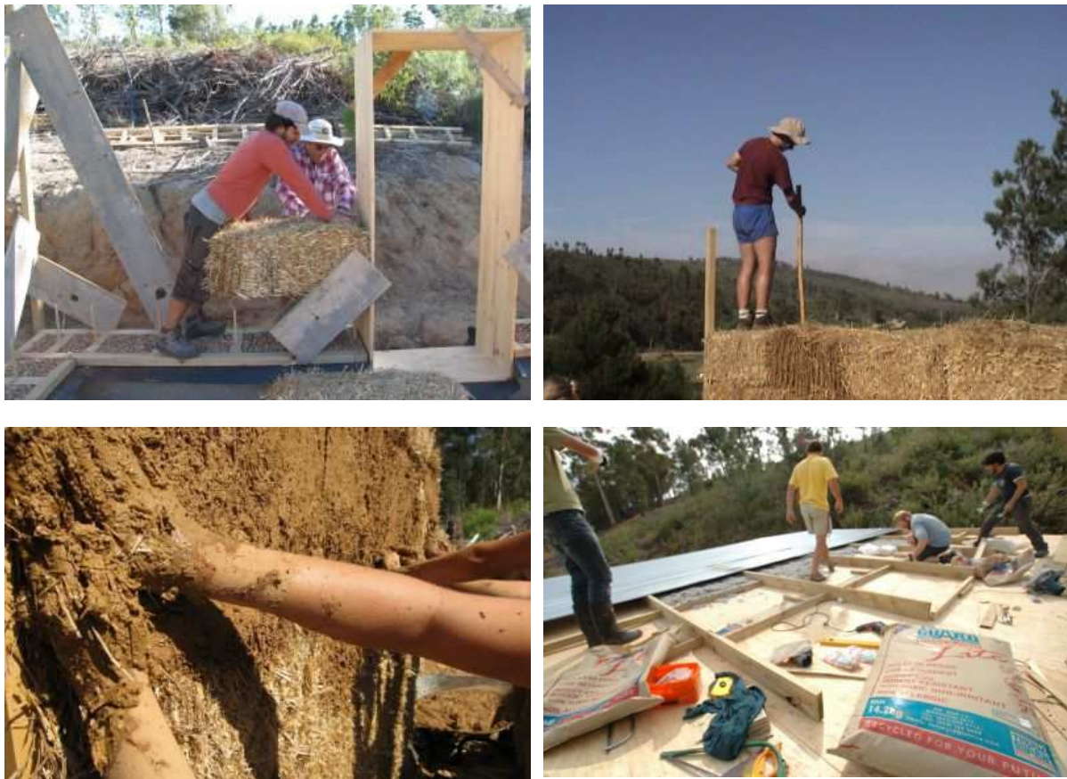
Top left: setting the first bale; top right: hammering a stake through the bales; bottom left: clay plaster on Straw Bale wall; bottom right: roof construction with Thermguard insulation
