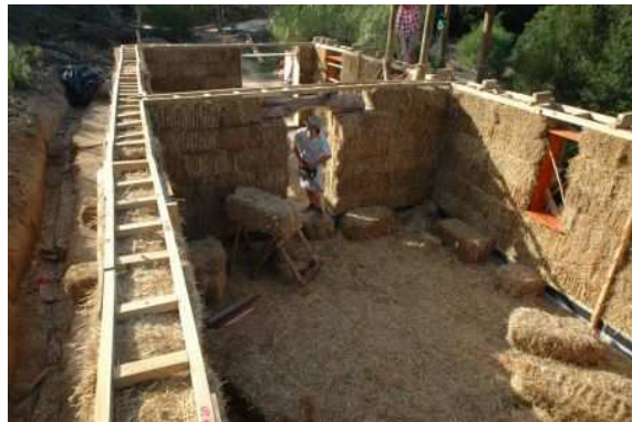
Fixing the wall plate to the bales
