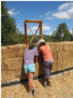
Wire tie-down system with wire stainer
