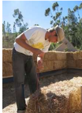
Making “pointies” out of blue gum stakes
