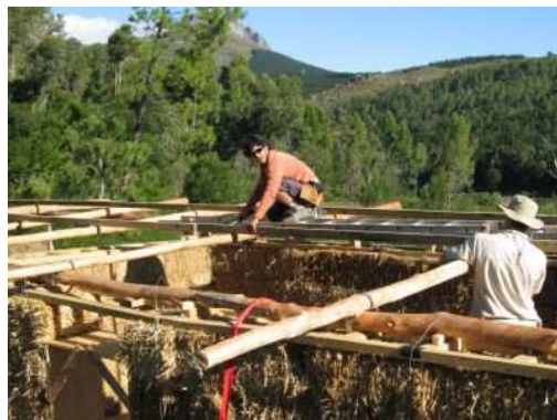
Fixing the roof beams
