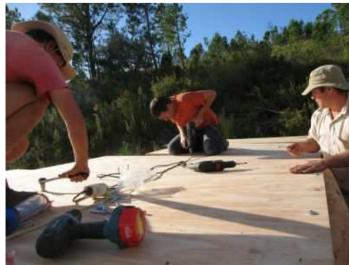
Laying a 100mm layer of recycled paper
