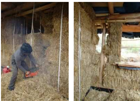
Taking out the rotting bales
