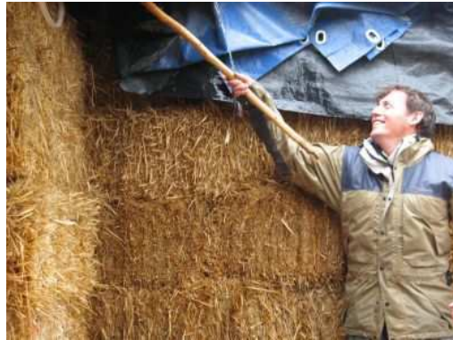
Damaged bales, rain came from top, travelled down along stakes, rotting quickly started
