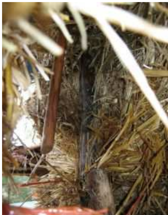
Damaged bales, rain came from top, travelled down along stakes, rotting quickly started
