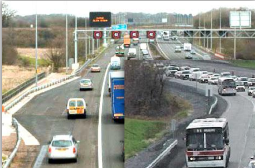
Temporary use of hard shoulder
