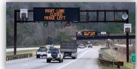
Lane control signals
